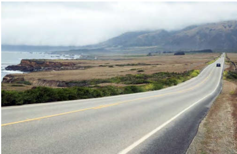
Figure 5-41 Low-lying Portions of Highway 1 in San Luis Obispo County
