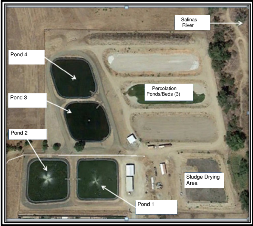
Figure 8. Current San Miguel WWTP
