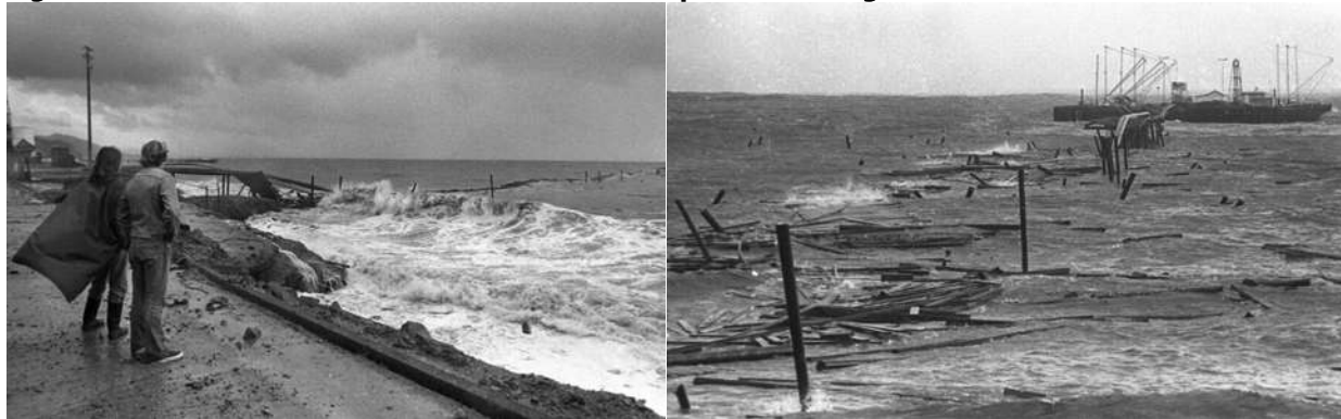
Figure 5- 36 Union Oil Pier in Avila Beach Collapses Following Severe 1983 Storm
