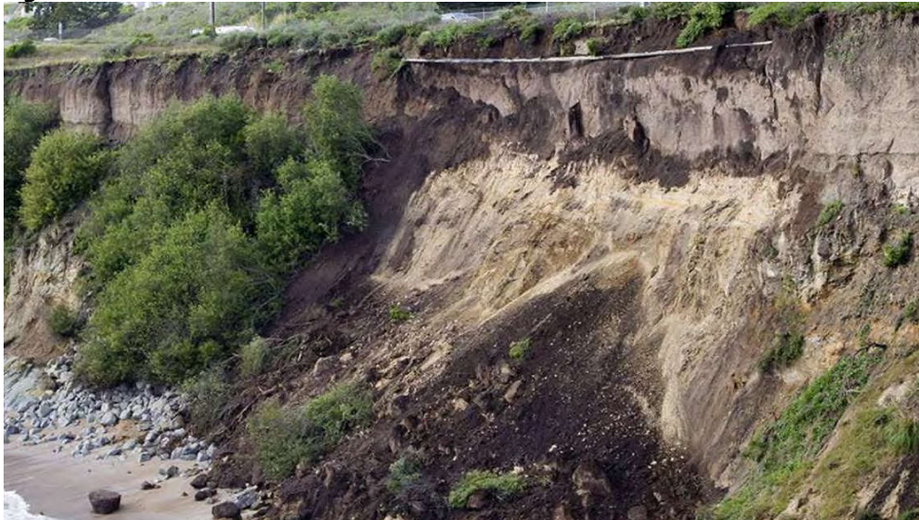
An approximate 100-foot section of cliff collapsed in Pismo Beach due to erosion of the bluff following winter storms in March 2011, demonstrating the severe impacts of coastal hazards on weak bluff sediments. Source: San Luis Obispo Tribune 2011
