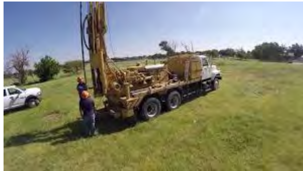
Truck-mounted HSA drilling rig
