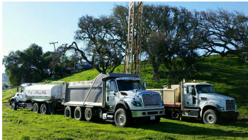
Rotary Water Well Drilling Equipment: Filipponi & Thompson Drilling
