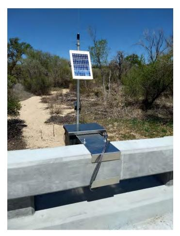
Figure 4. Creston (Huer Huero Creek) radar sensor stream gage installation
