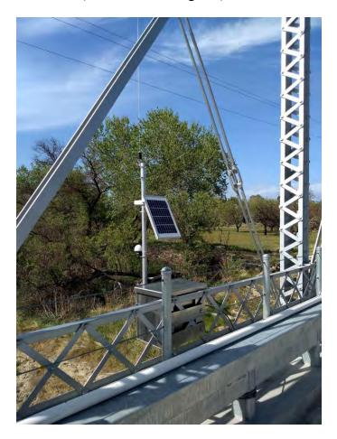
Figure 2. Whitley Gardens (Estrella River) radar sensor stream gage installation
