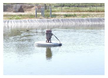
Figure 4.3. Surface Mechanical Turbine Aerator in Pond 1
