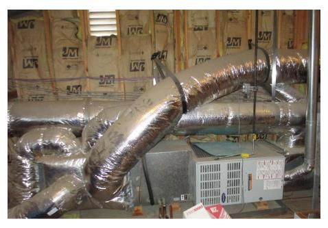
Figure 2.12: Carrier 6-ton Air Handler in Attic of District Office
