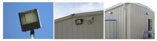
Figure 4.2. WWTP HPS (left), WWTP MH wall pack (center), Well pump 4 MH wall packs (right)
