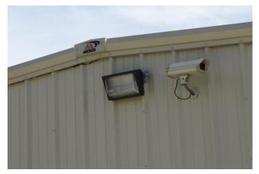
Figure 2.11: Typical MH Wallpack at Well Pump Station
