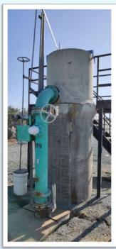
Float valve style turnout Supports better operations and system safety
